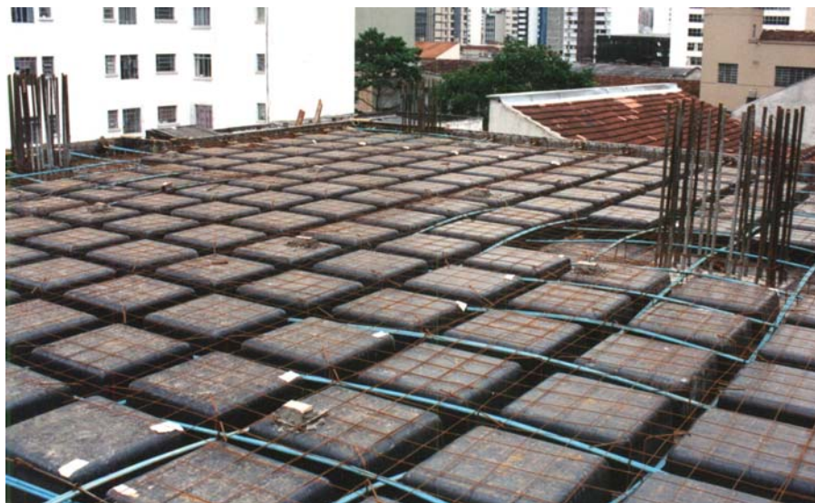
FIGURE 2 POST-TENSIONED WAFFLE SLAB
